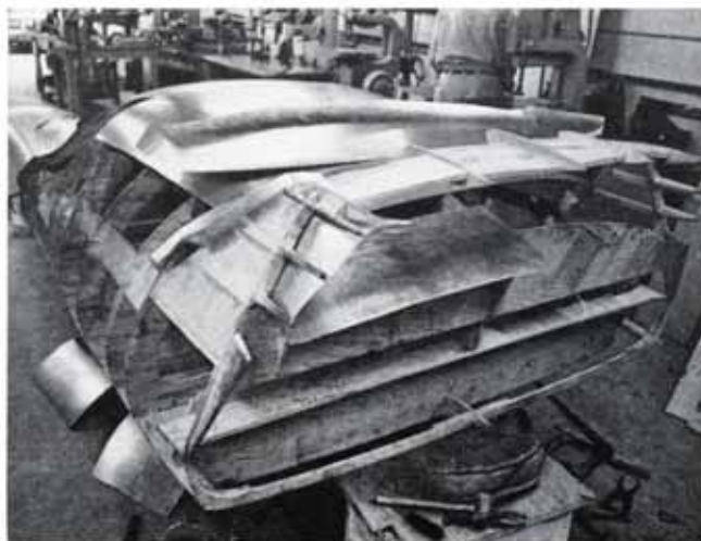
Aluminum takes shape over plywood forms at T-B.
